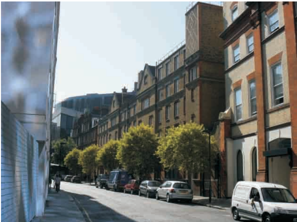
Plate 2: Parker House frontage viewed from the east
