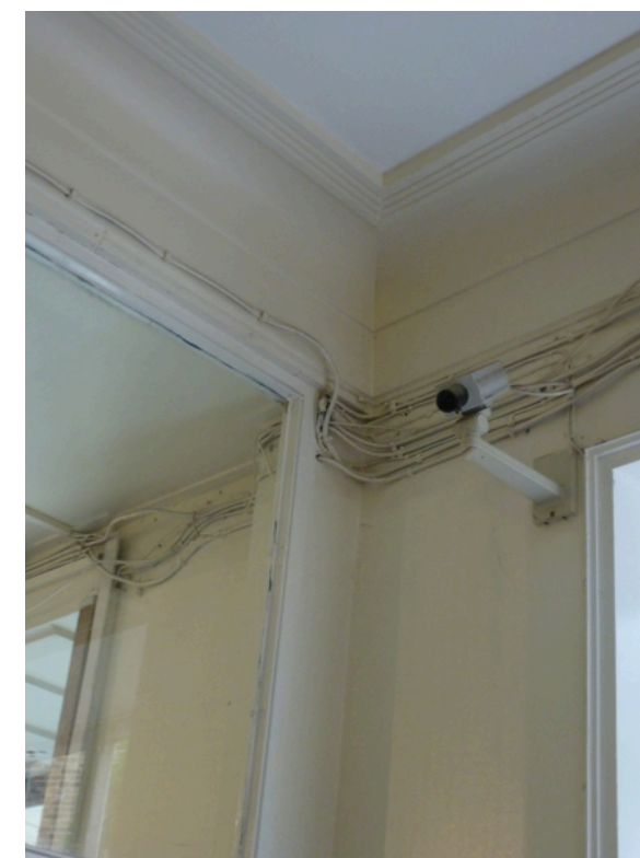
B SURFACE WIRING INSTALLATION
