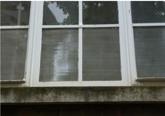
existing crittall steel windows retained, new doorway to match
