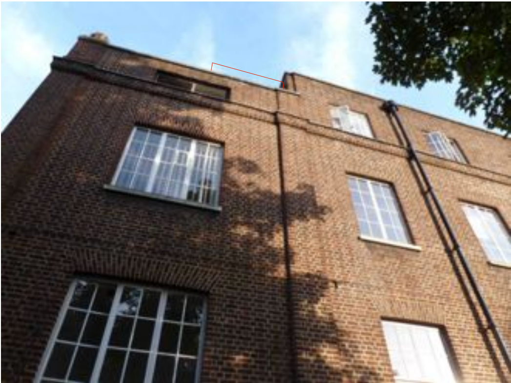
external view of lift overrun, curtains to obscure portion of lift shaft seen through existing windows
