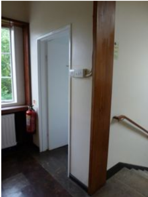
doorway to existing stair lobby retained
