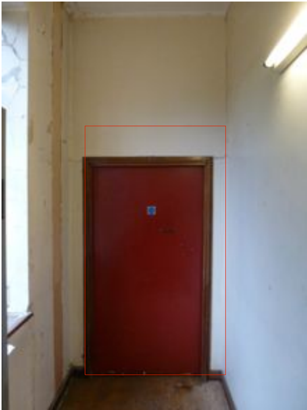
reconfiguration of existing dor to suit lift door
