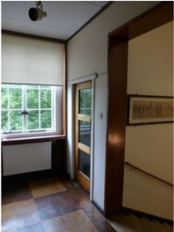
doorway to existing stair lobby retained
