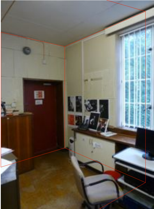
demolition of floor /Ceiling and construction of shaft walls
