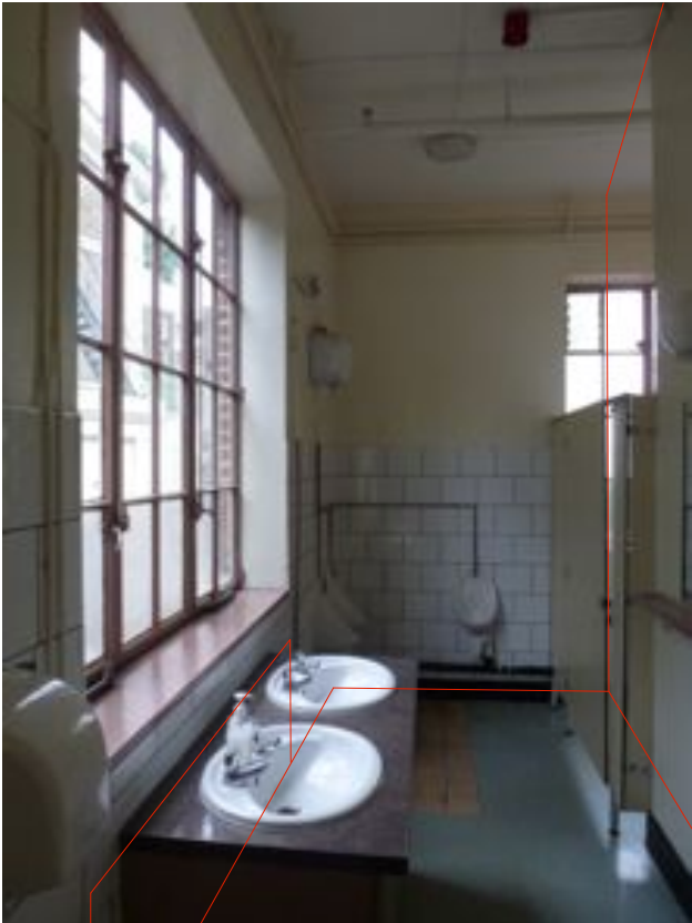
demolition of floor and below window for entry + new wall
