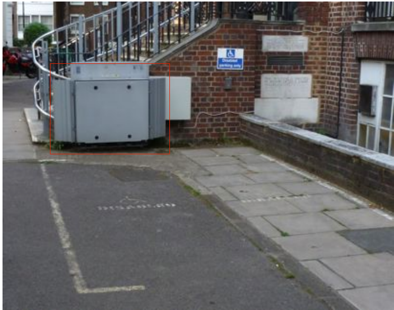
existing stair lift and rails removed
