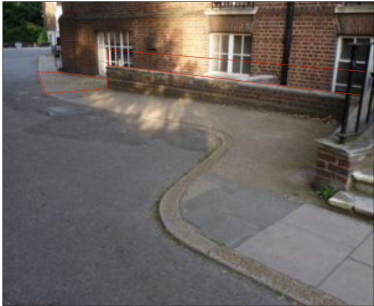
external concrete removed and relaid at new entrance thershold location of new railings indicated in retained parapet wall
