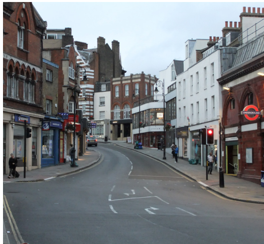
View from outside Hampstead underground station
