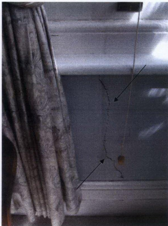
2mm Vertical/Diagonal cracking below bay window at ground floor level.
