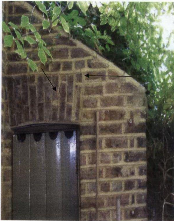
3mm Stepped cracking in brickwork above the door.
