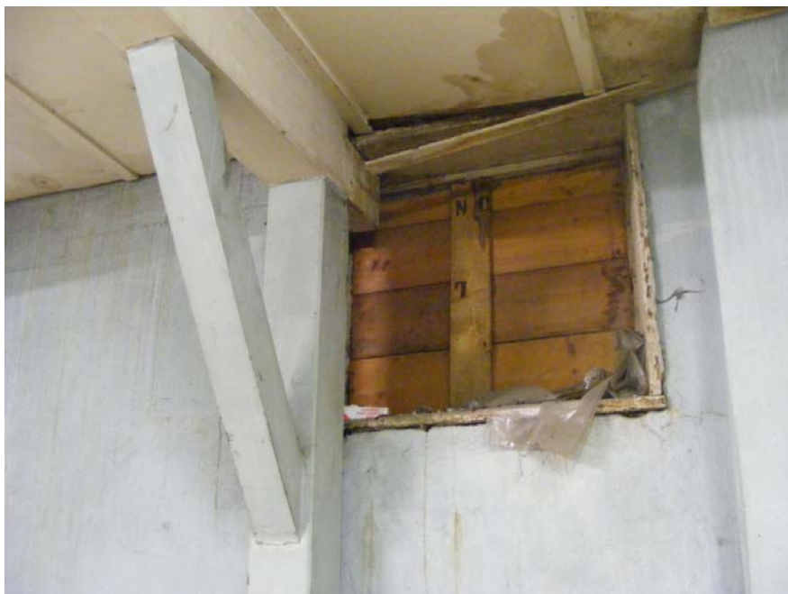
Plate 12: Ground floor – blocked opening in rear wall
