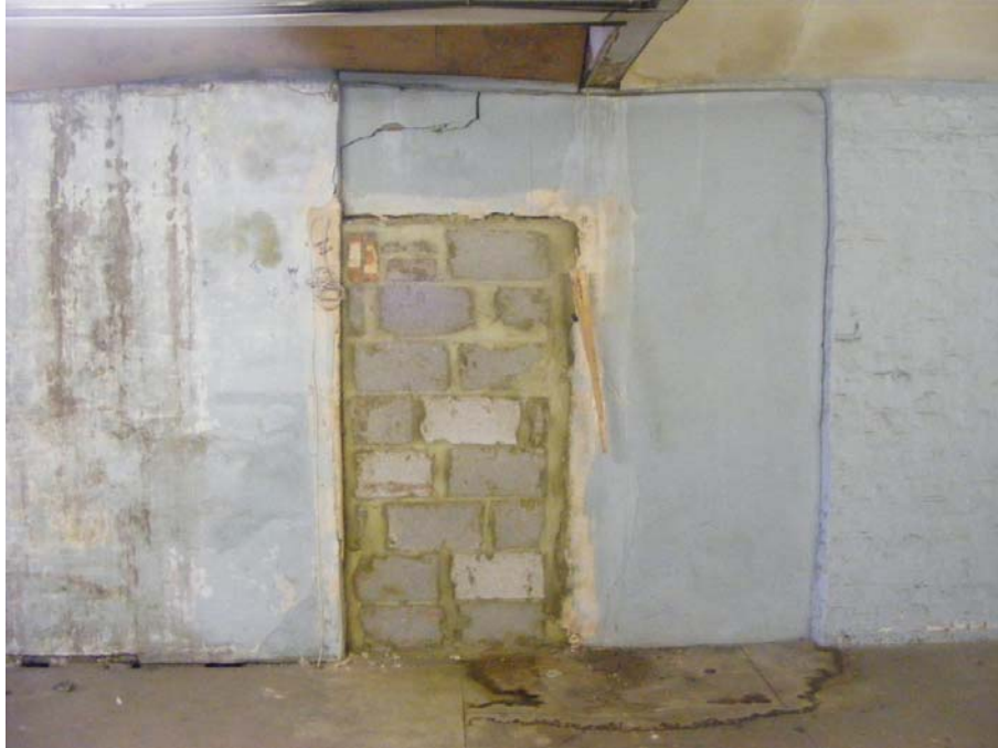
Plate 15: Blocked internal doorway to 21 King's Mews, first floor
