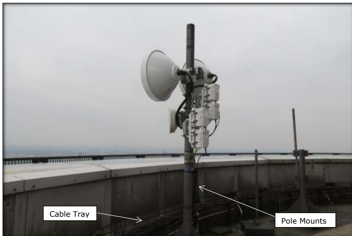
Plate 1: Example of fixing and cable run on top of the advertising section of the BT Tower. (R4 Telecom, 2012)
