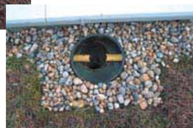
Bauder inspection chamber with surrounding pebble vegetation barrier.
