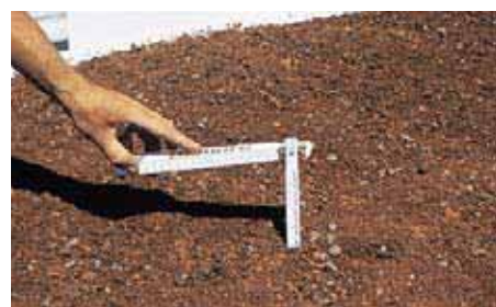
Measuring the correct depth of growing medium.
