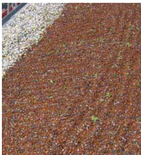
Seeds and plant cuttings spray applied to recently prepared substrate growing medium.
