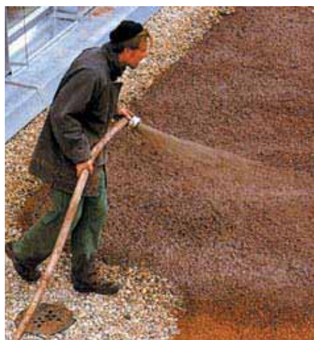
Applying the special spray mix to the substrate growing medium.
