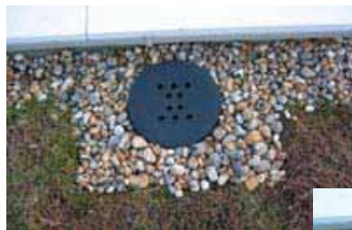
Bauder inspection chamber with surrounding pebble vegetation barrier.
