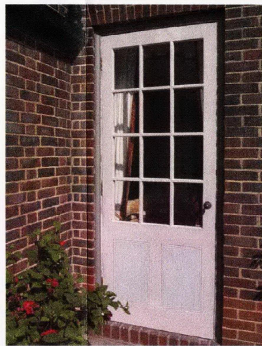
WHITE PAINTED SINGLE LEAF TIMBER DOOR, TO MATCH EXISTING WINDOW, WITH FIXED WINDOW ABOVE AND SOLID PANEL BELOW AS REQUESTED (SEE MATERIAL SAMPLE 05)
