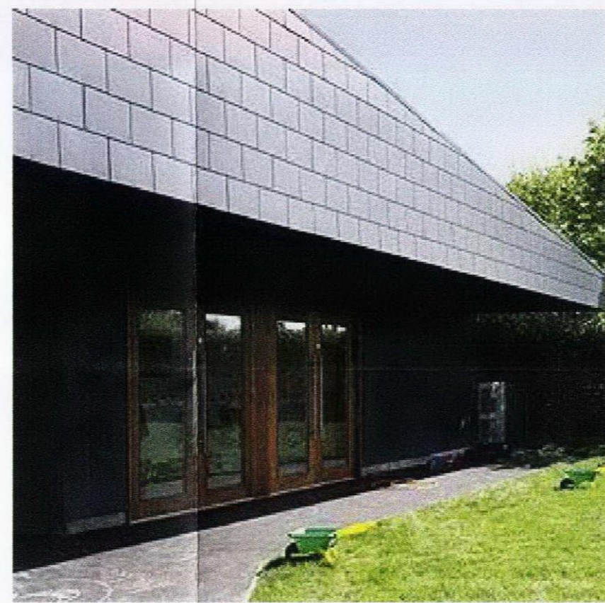
ENGINEERED SLATE CLADDING (MARLEY ETERNITE) (SEE MATERIAL SAMPLE 03)
