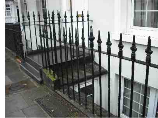
Photograph of the front lightwell to the Basement
