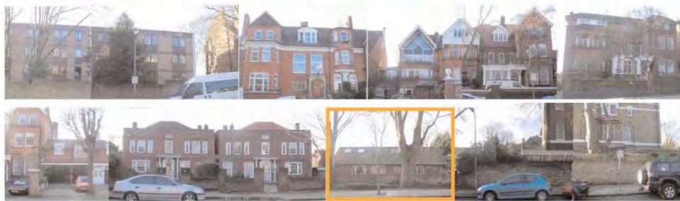
West side of Maresfield Gardens with 55, 57 and 59 highlighted. Streetscape is made up of a variety of scales and styles, with a number of buildings showing a variety of scales and styles within themselves
