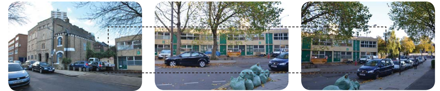
Existing workshops to be demolished
