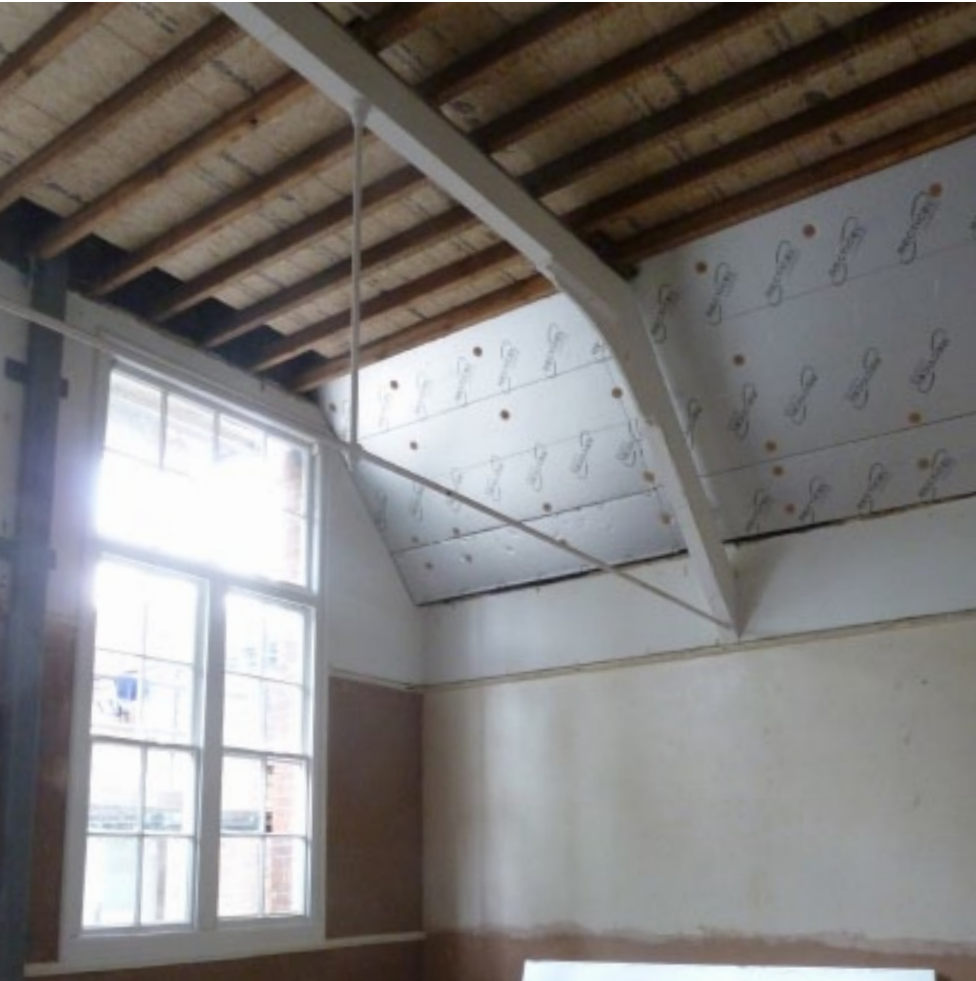
Completed and Construction photographs of Robert FitzRoy Academy, Croydon by Architype. The original ceilings were removed which allowed them to be insulated and have acoustic treatments applied - a similar strategy to that proposed for CCfL.
