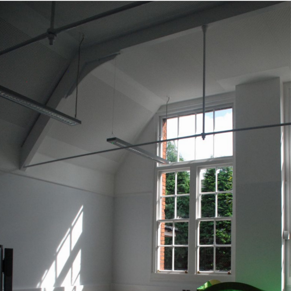
Completed and Construction photographs of Robert FitzRoy Academy, Croydon by Architype. The original ceilings were removed which allowed them to be insulated and have acoustic treatments applied - a similar strategy to that proposed for CCfL.
