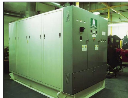
Energy flow of CHP compared to conventional provision of heat and power & typical small scale CHP engine located in plant room (Source: GPG388: Combined Heat and Power for Buildings, Action Energy).
