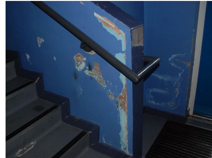
Damp damage in 2002 building
