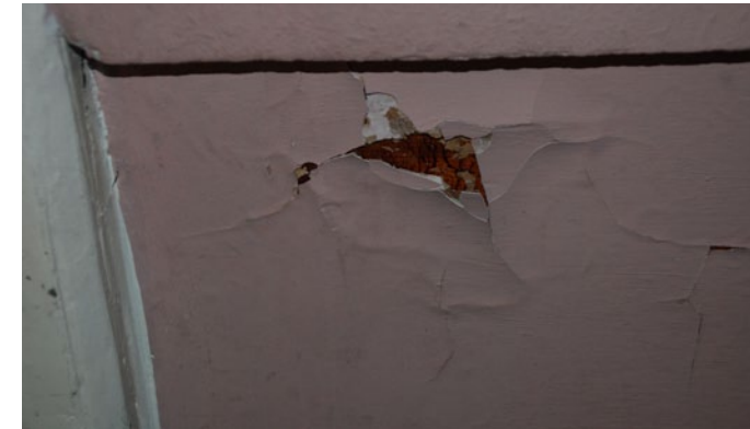
Water ingress damage in original building
