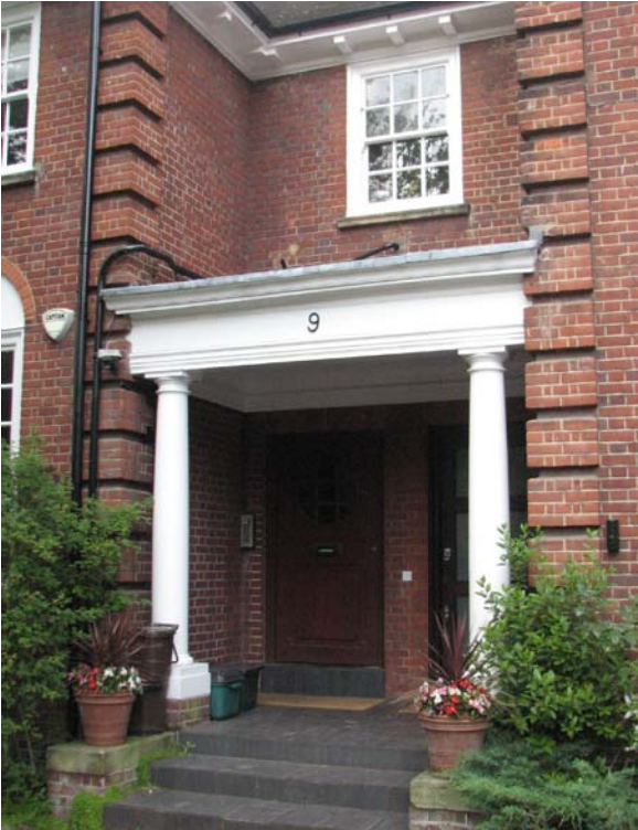
EXISTING FRONT ENTRANCE PH-01
