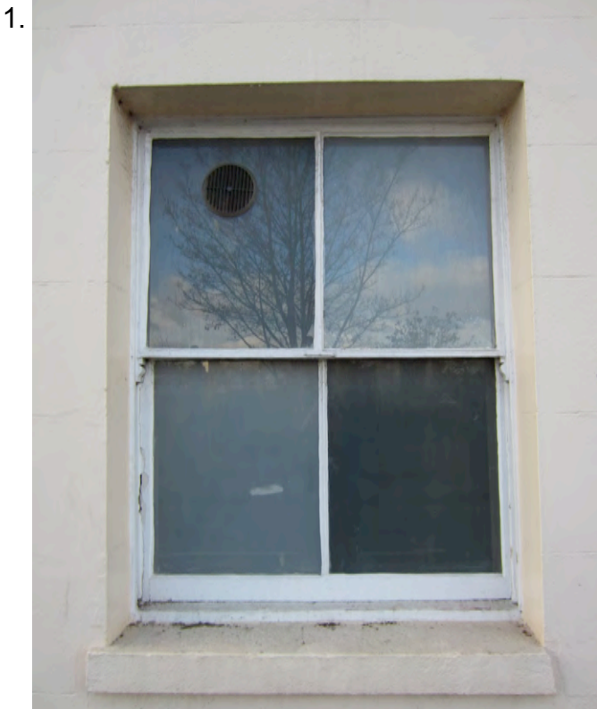
This original window opening has been repaired with replacement sashes fitted. The glazing bars are heavier in profile and do not align, the horns do not match the originals, obscure glass has been installed (including a bathroom extract fan). The windows in not in keeping with the original details. Proposal to replace with new historic single glazed window to match original details.
