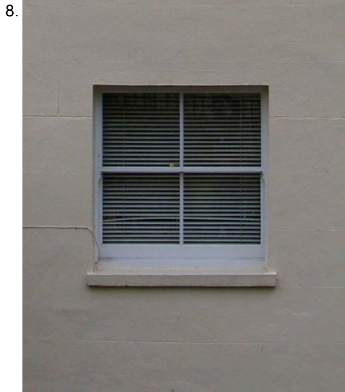
Non-original opening (post 1955). This window is to be replaced with an arched door as previous approved application 2011/1435/L
