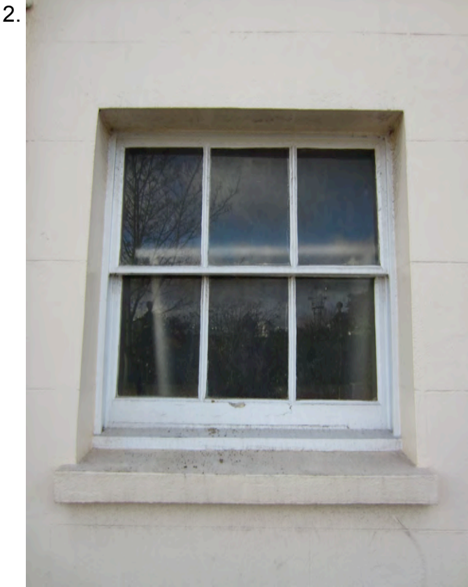
Non-original opening (post 1955). Window sashes and glazing bars are heavier, no horns and generally not in keeping with historic details. Proposal is to replace with new historic single glazed window to match original details.
