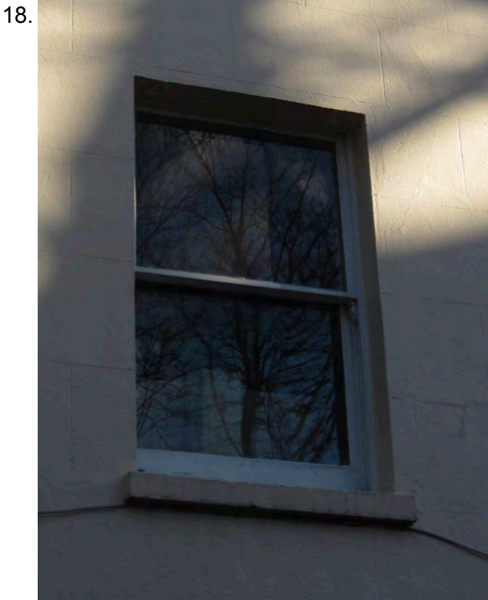
Non-original rear window (added post 1955). No glazing bar, not in keeping with other windows. This window is to be replaced with new glazed doors as per previous approved application 2011/1435/L.
