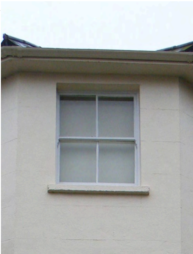
Original window has been repaired and partially replaced over time. In poor condition, glazing bars don't line up & there is also a large gap between sashes. Proposal is to replace with new conservation double glazed sash window to traditional details.
