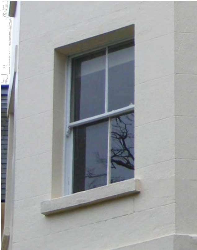
Original window has been repaired and partially replaced over time. Bottom sash has heavier glazing bar & thicker window frame than the original windows (see detail 14a). There is also a large gap between sashes (similar to detail 16a). Proposal is to replace with new conservation double glazed sash window to traditional details.
