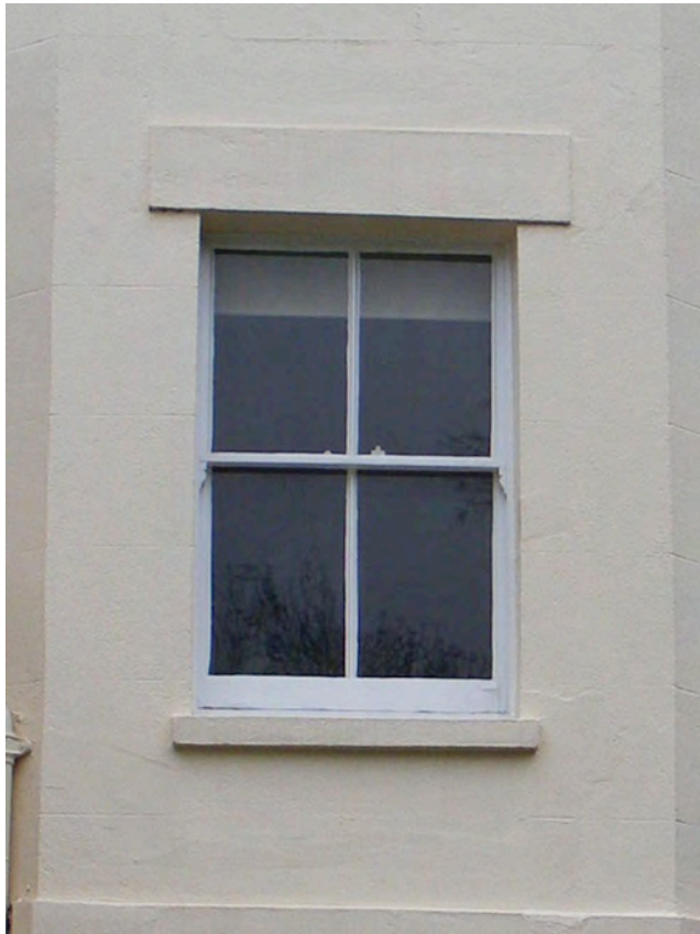
Original window has been repaired and partially replaced over time. Both sashes have heavier glazing bars than the original windows. Proposal is to replace with new conservation double glazed sash window to traditional details.
