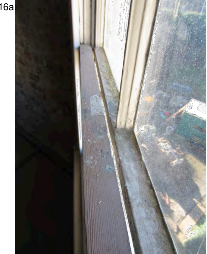
Internal detail of window 16 shows the window in a poor state of repair & the large gap between the two poorly constructed sashes.
