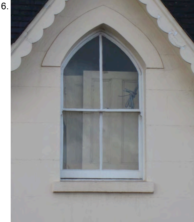
Original window has been repaired & partially replaced with non original sash and is generally in poor condition. Top sash has heavier glazing bar. Proposal to replace with new single glazed window to match original details.
