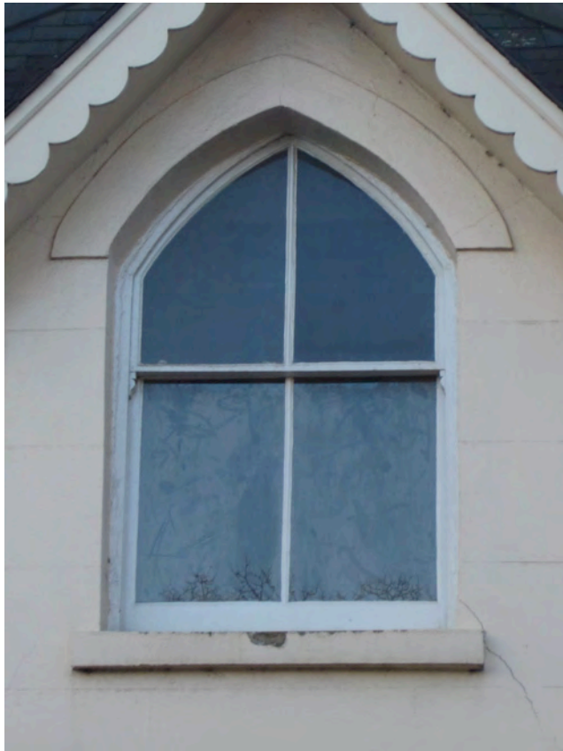
Non-original opening (post 1955). Window sashes and glazing bars are heavier and generally not in keeping with historic details. Propose to replace with new single glazed sash window to match historic details.
