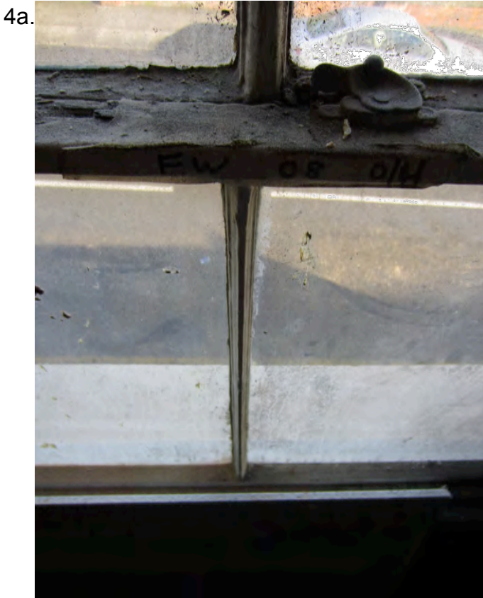
Internal detail of window 4. Note the glazing bars do not align. The bottom sash is original but in a poor state of repair this has an 18mm glazing bar, the upper sash is a replacement with heavier glazing bar at 23mm.
