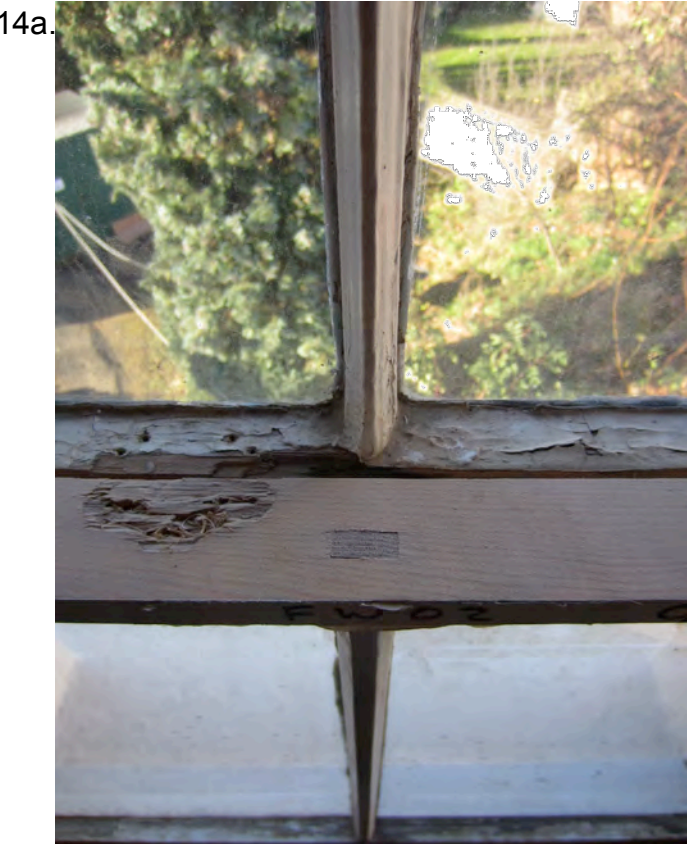
Internal detail of window 14 shows the window in a poor state of repair & different glazing bar details for the top & bottom sashes. Also the more recently installed bottom sash is deeper than the top sash.
