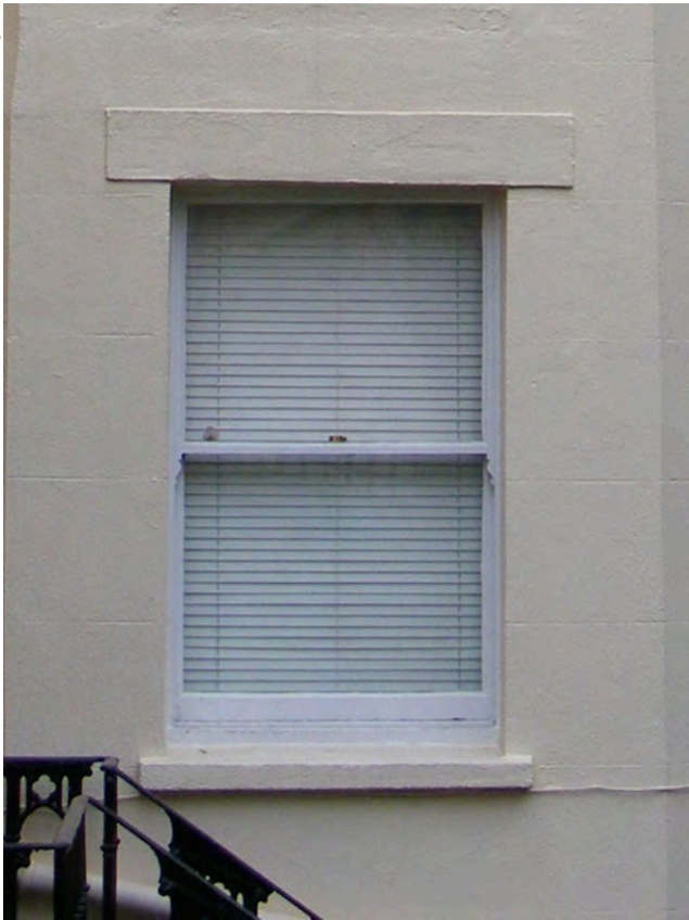
Non-original window (post 1955). Most likely added when rear elevation windows were fitted after 1955. No glazing bar, not in keeping with other windows. Proposal is to replace with new conservation double glazed sash window to traditional details.
