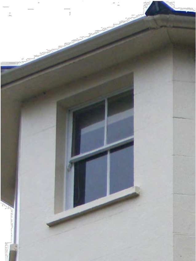
Original window has been repaired and partially replaced over time. In poor condition & there is a large gap between sashes (see detail 16a). Proposal is to replace with new conservation double glazed sash window to traditional details.
