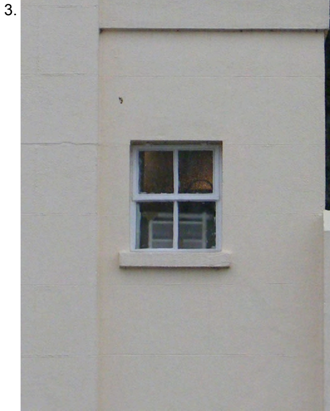
Non-original opening (post 1955). Window sashes and glazing bars are heavier, no horns and generally not in keeping with historic details. This window is removed and infilled as previous approved application 2011/1435/L
