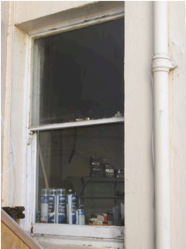
Non-original window (post 1955). Most likely added when rear windows were fitted after 1955. No glazing bar, not in keeping with other windows. Proposal is to replace with new conservation double glazed sash window to traditional details.
