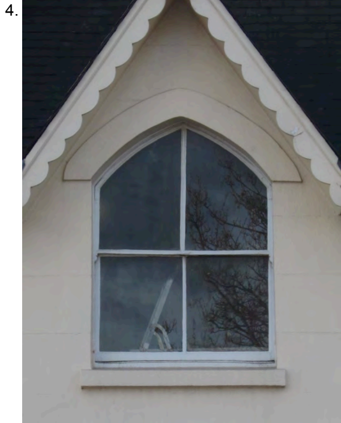
This original window has been repaired and partially replaced with non original sash fitted (circa 1955). The glazing bars no not align (see 4a detail photograph). The horns do not match on either side, and the window is generally in poor condition. Proposal to replace with new historic single glazed window to match original details.
