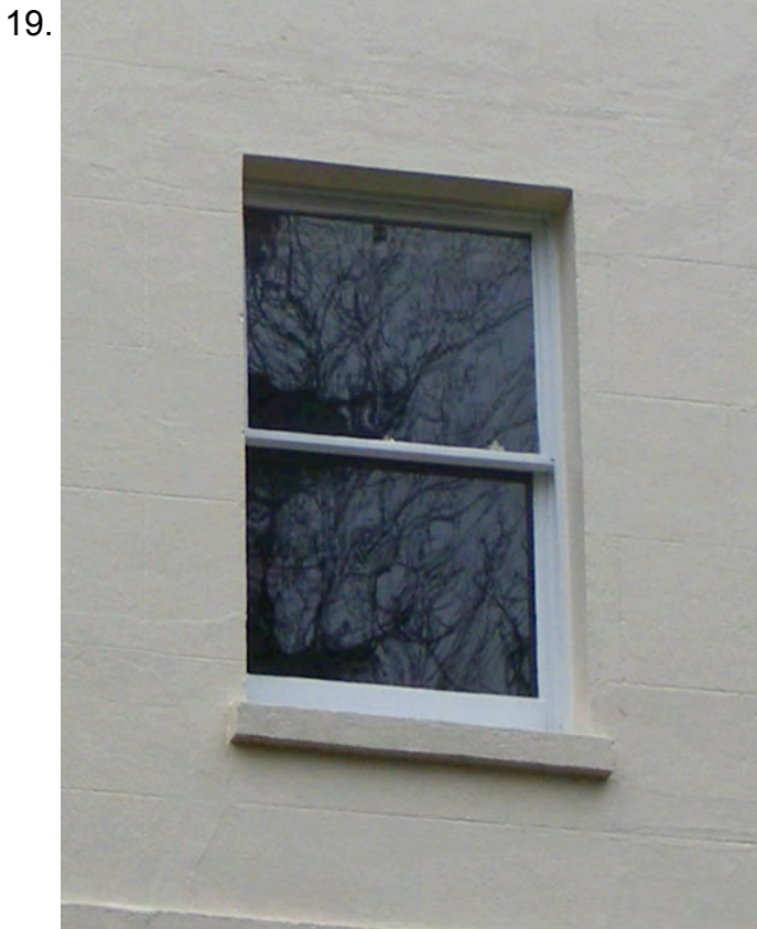
Non-original rear window (added post 1955). No glazing bar, not in keeping with other windows. New wider window to be added as per previous approved application 2011/1435/L. Proposal to replace with new conservation double glazed sash window to traditional details.
