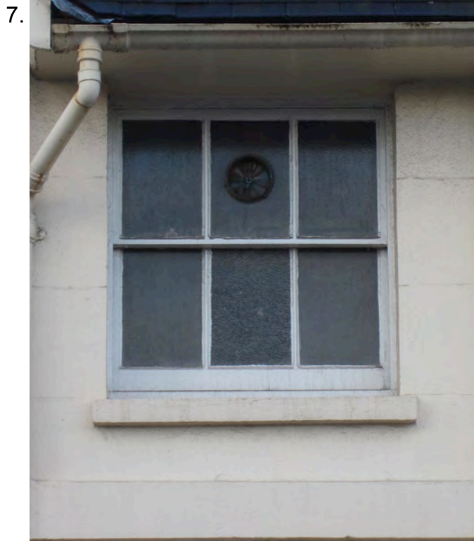
Non-original opening (post 1955). Window sashes and glazing bars are heavier, no horns, obscure glass has been installed (including a bathroom fan). Generally not in keeping with historic details. Proposal is to replace with new single glazed window to match original details.
