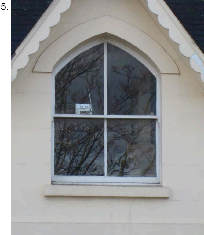
Original window has been repaired & partially replaced with non original sash. The window is generally in poor condition. Proposal to replace with new single glazed window to match original details.
