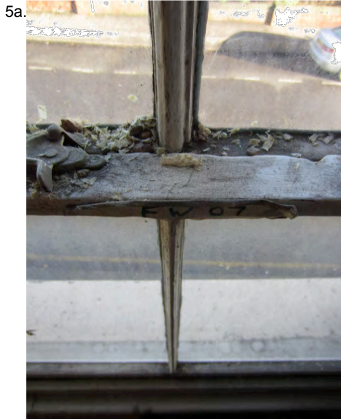
Internal detail of window 5 shows the window in a poor state of repair, with different glazing bar profiles for the top & bottom sashes again.
