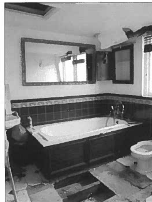
ROOM [202] Existing floor
