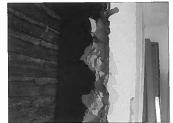
Investigation Work: Photograph showing 1 layer of plasterboards fixed to studwork. (photo taken from room 2.01)
