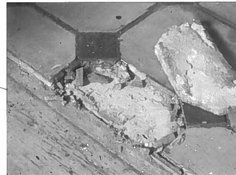
Photograph showing the existing substrate under tiles in G.03. modern plywood is laid under the tiles.
