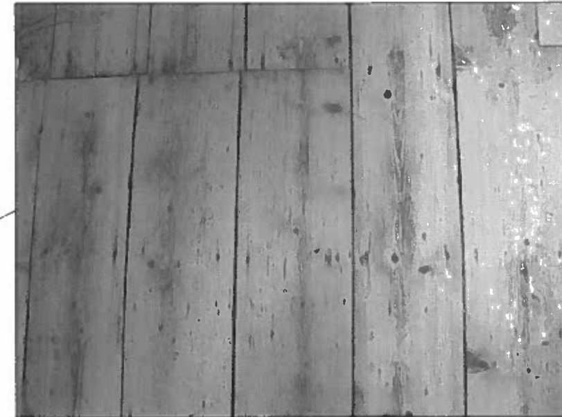
Photograph showing the existing SW boards in G.02. Same/similar floorboards are laid in rooms 1.01 and 2.01. They are approximately 20mm thick, widths between 190mm and 220mm.
