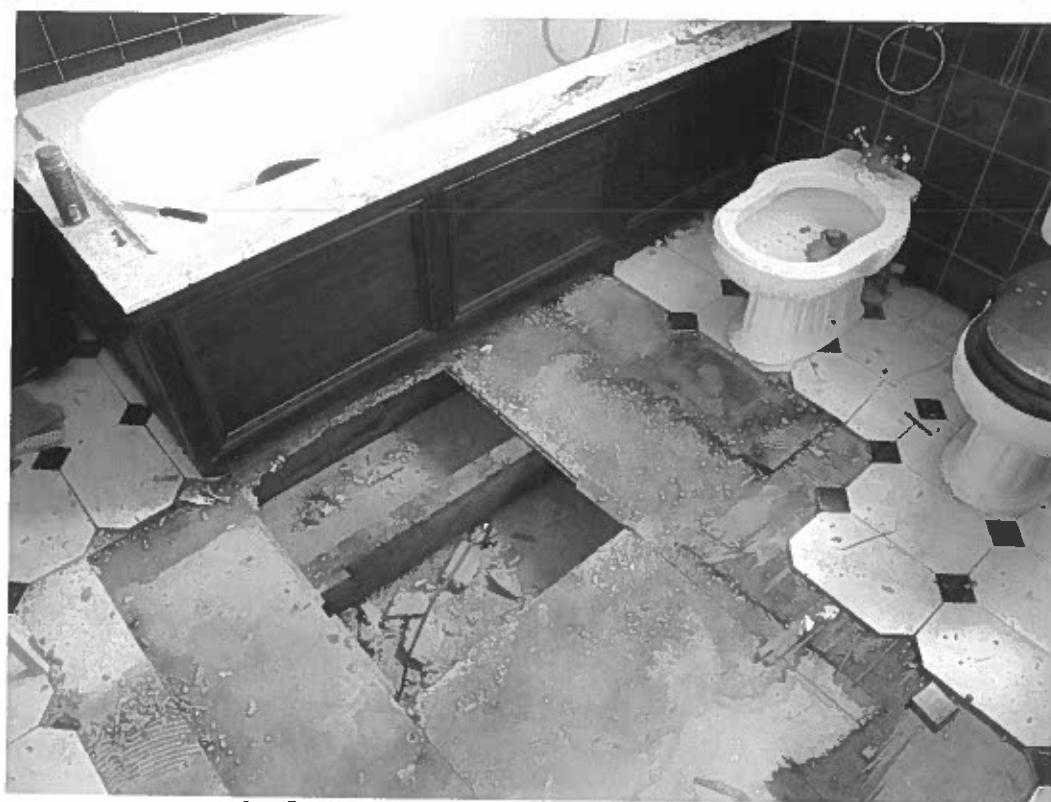
2. Second floor rear room. Joists to be doubled up
