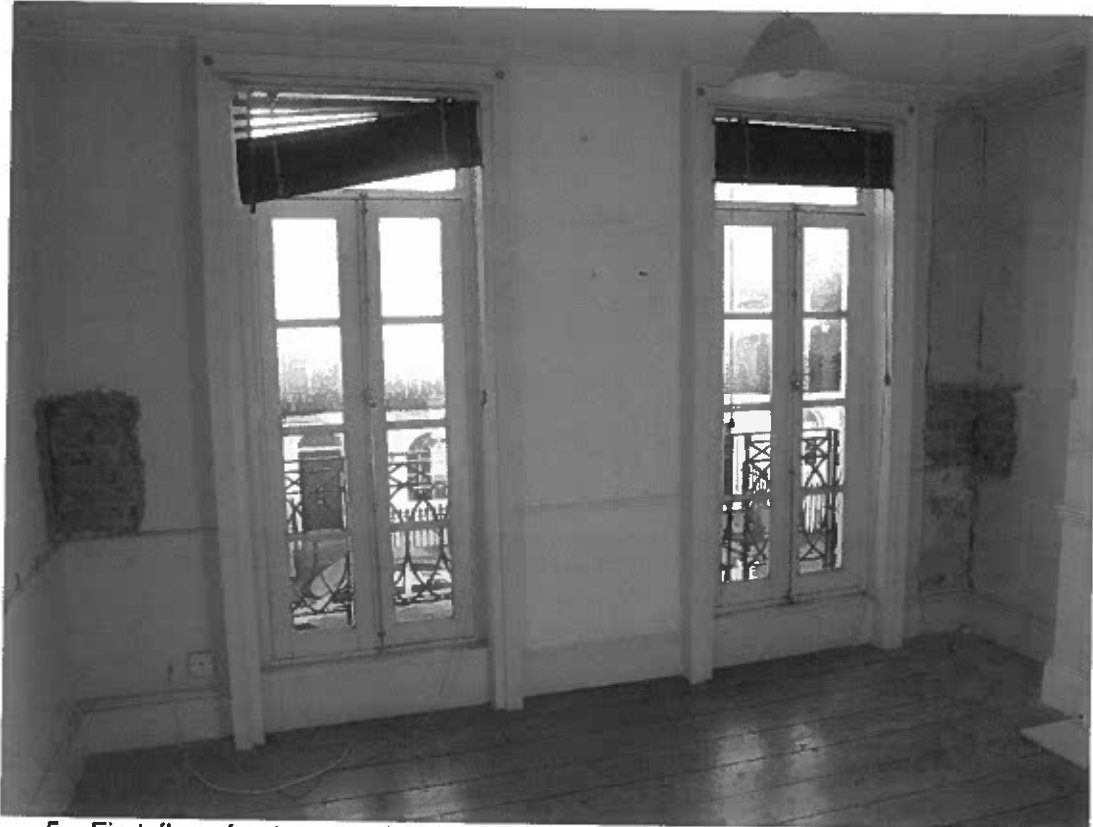
5. First floor front room showing opening up to expose bond between front and party walls
