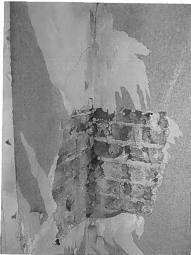
9. Second floor front wall. Poor bond to party wall 11/13
