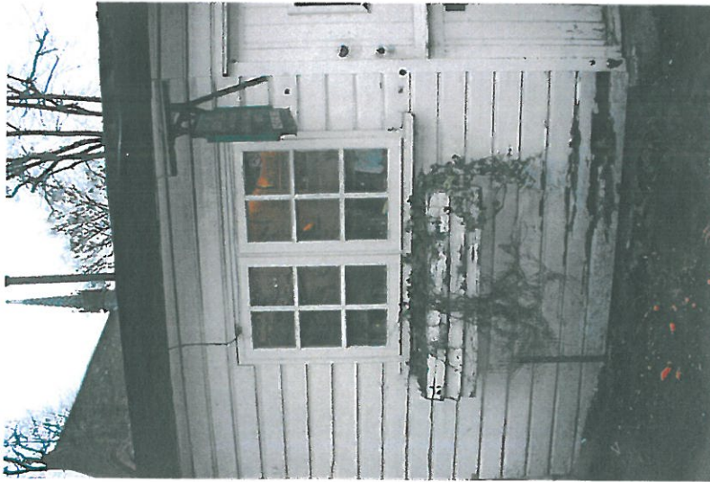
4. Clockmaker - Rotten weather boarding.
