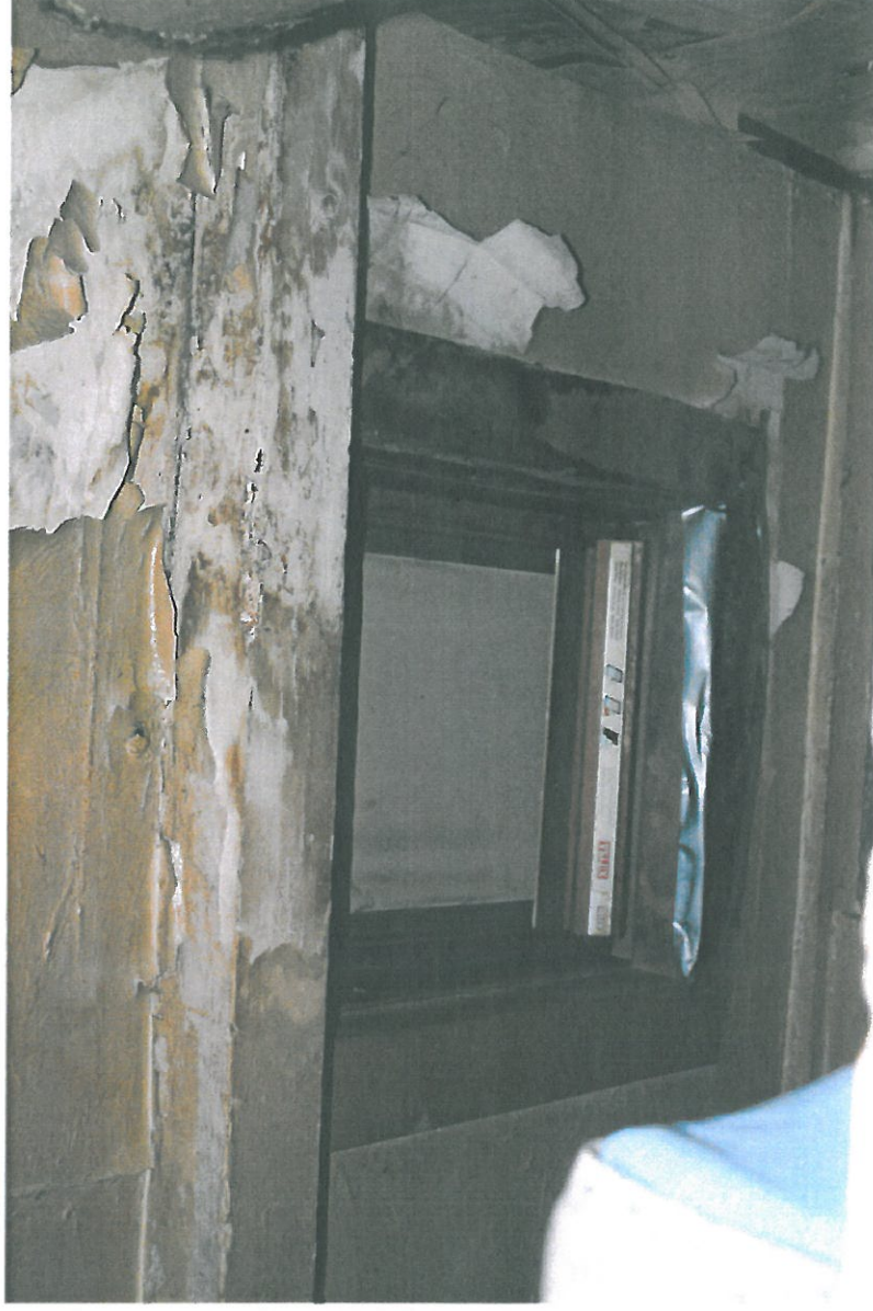
11. Studio - damp roof structure - velux roof light showing water penetration..
