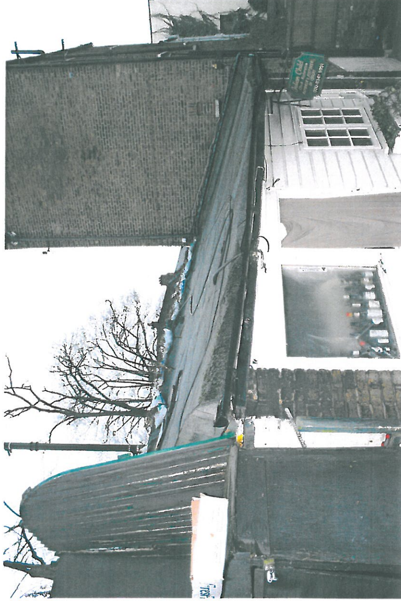
7. Exterior felt roof - poor condition.
