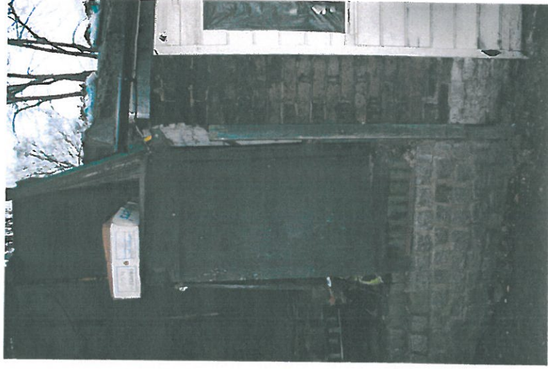
2. Studio - damp brickwork pier.
