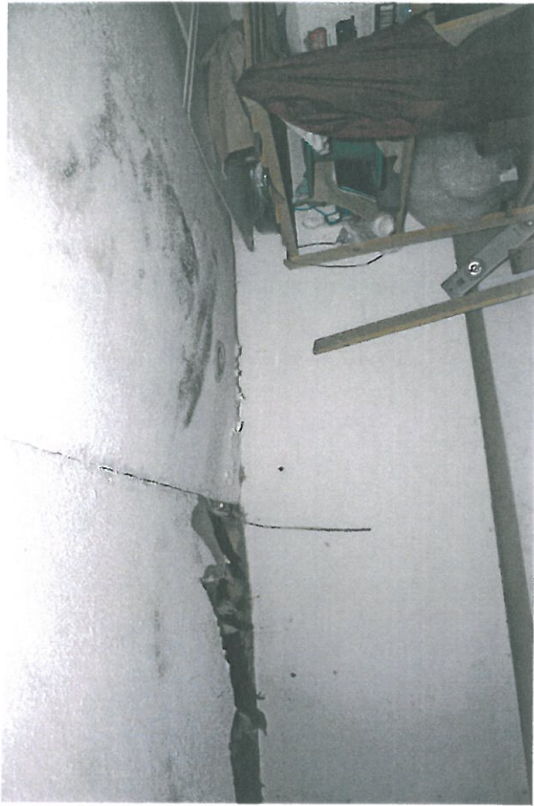
15. Snowhill Store - bowing damp ceiling.
