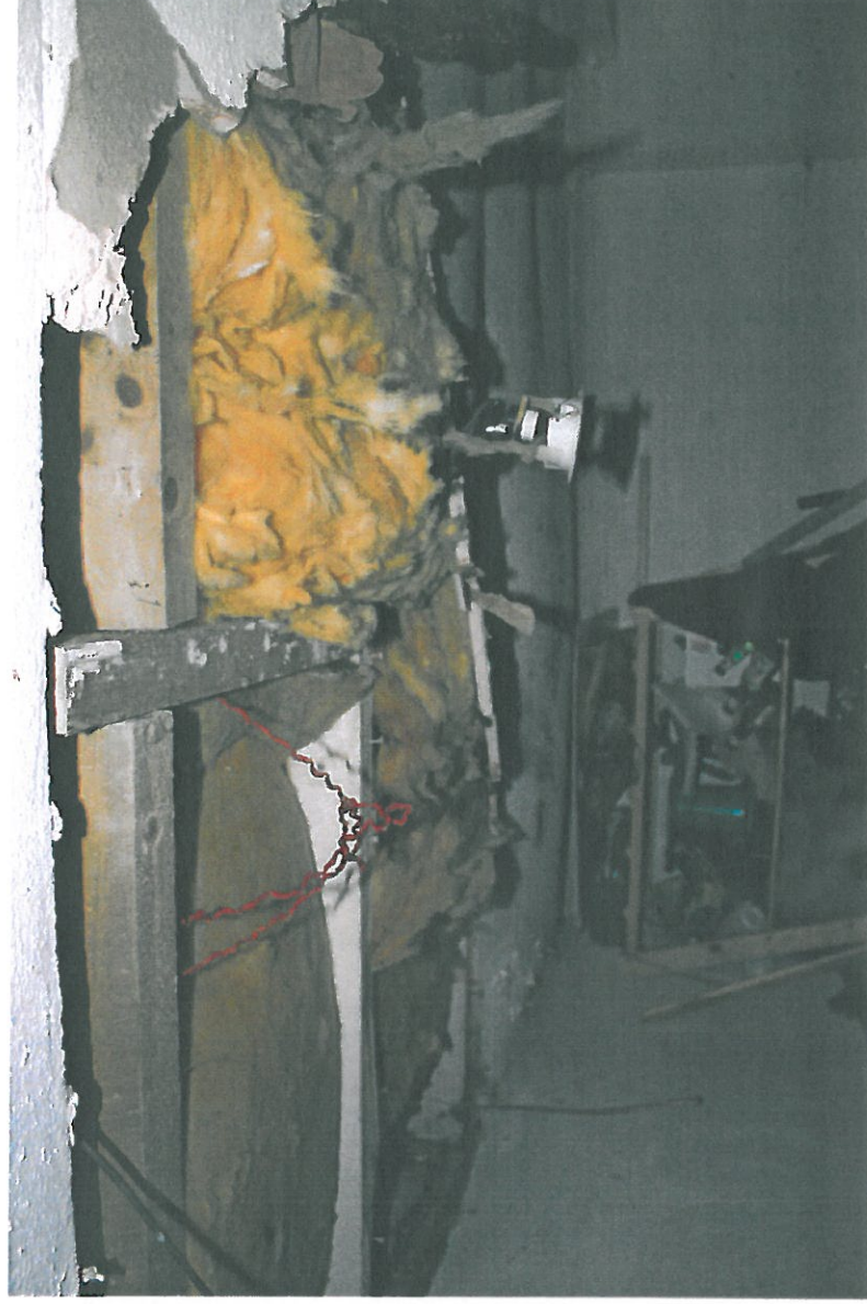
13. SnowHill Store - collapsed ceiling.
