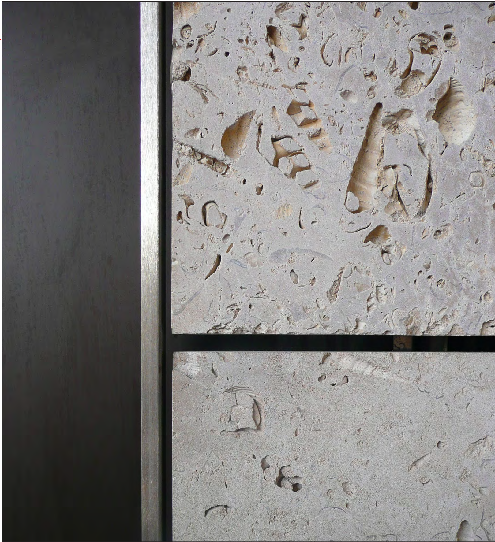
Fig. P070799 JORDANS ROACH LIMESTONE CLADDING EDGE DETAIL
