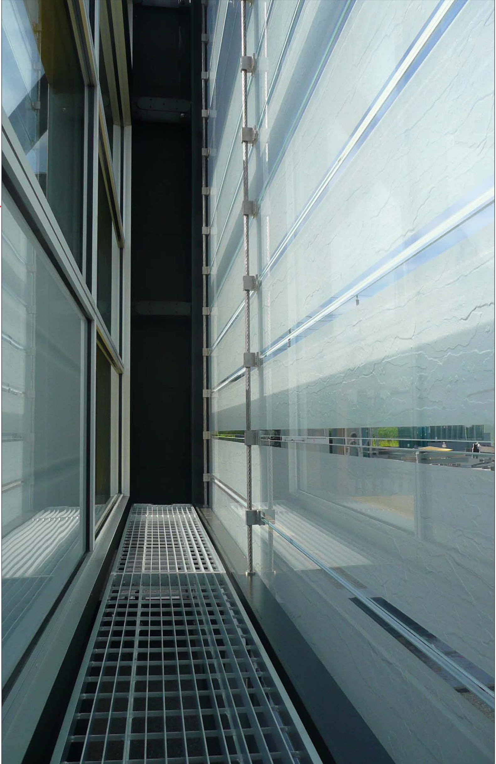
Fig P1070255 INTERIOR VIEW BETWEEN CAST GLASS AND DOUBLE GLAZED FACADE
