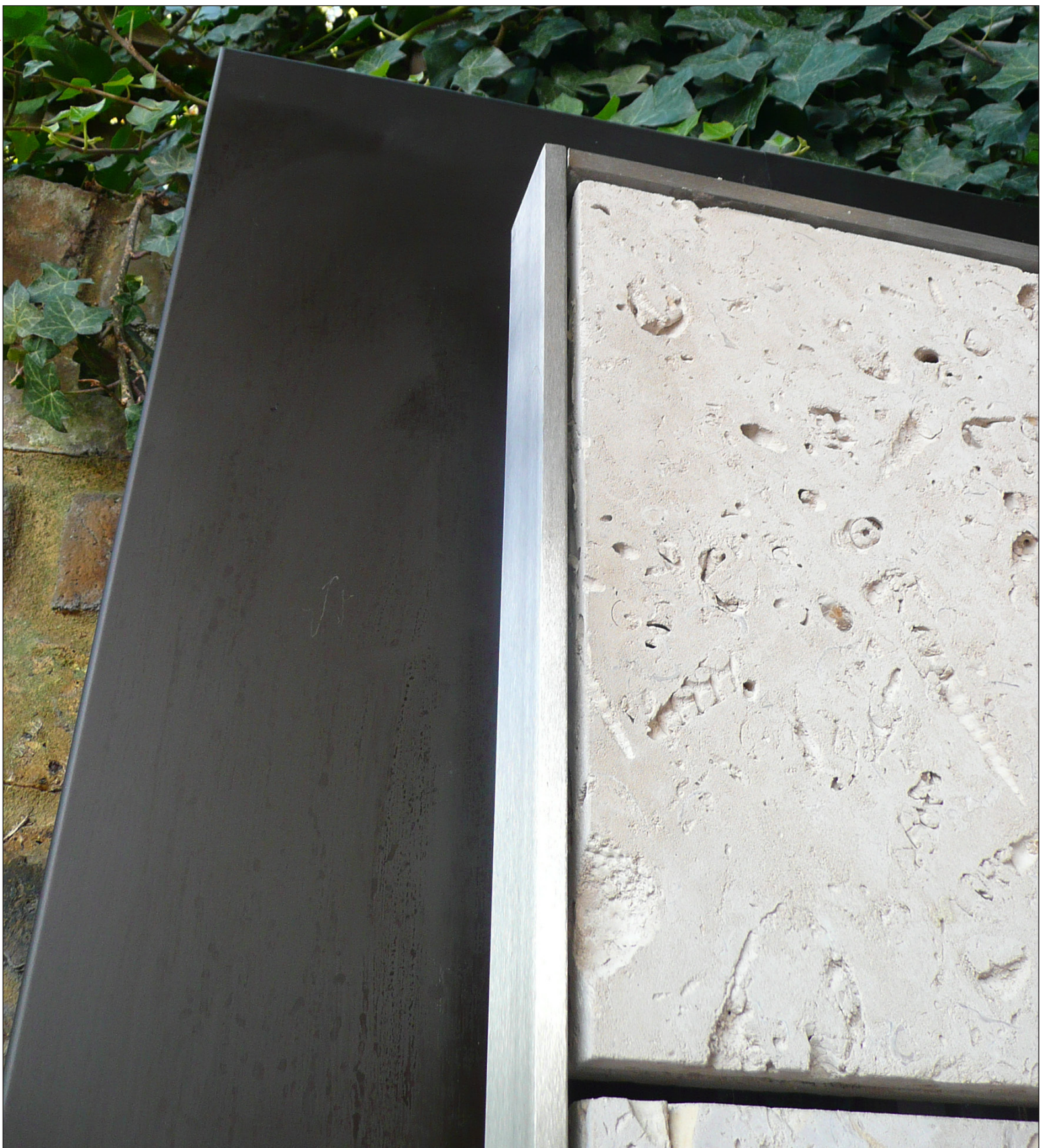
Fig P1070801 PORTLAND LIMESTONE CLADDING CORNER DETAIL
