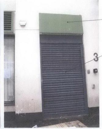
Existing metal fascia to be removed wall made good and prepared for canopy
