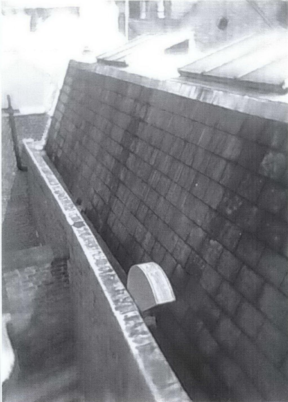
Roof 8-10 Neal's Yard .
