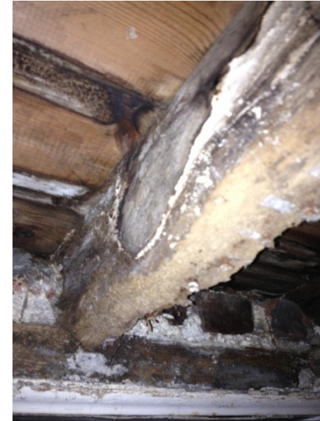
Wet rot on first floor joists
