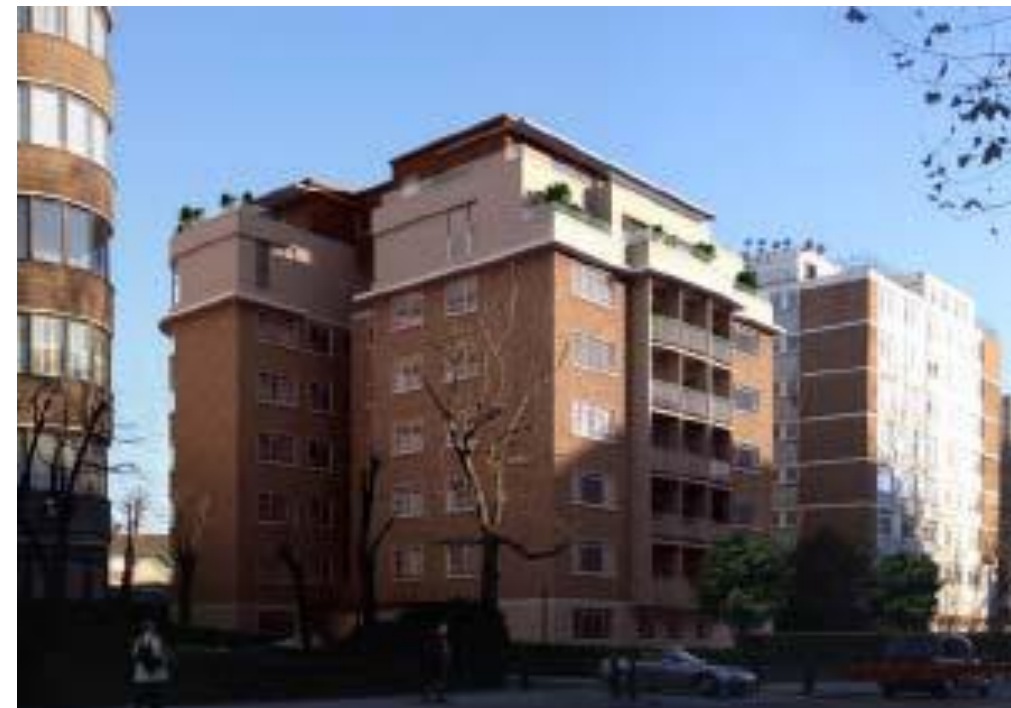
Typical approach to roof extension, St John's Wood
