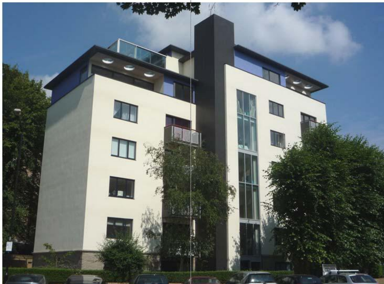
Pirton Ltd - before and after views, Parkland Court, Kensington
