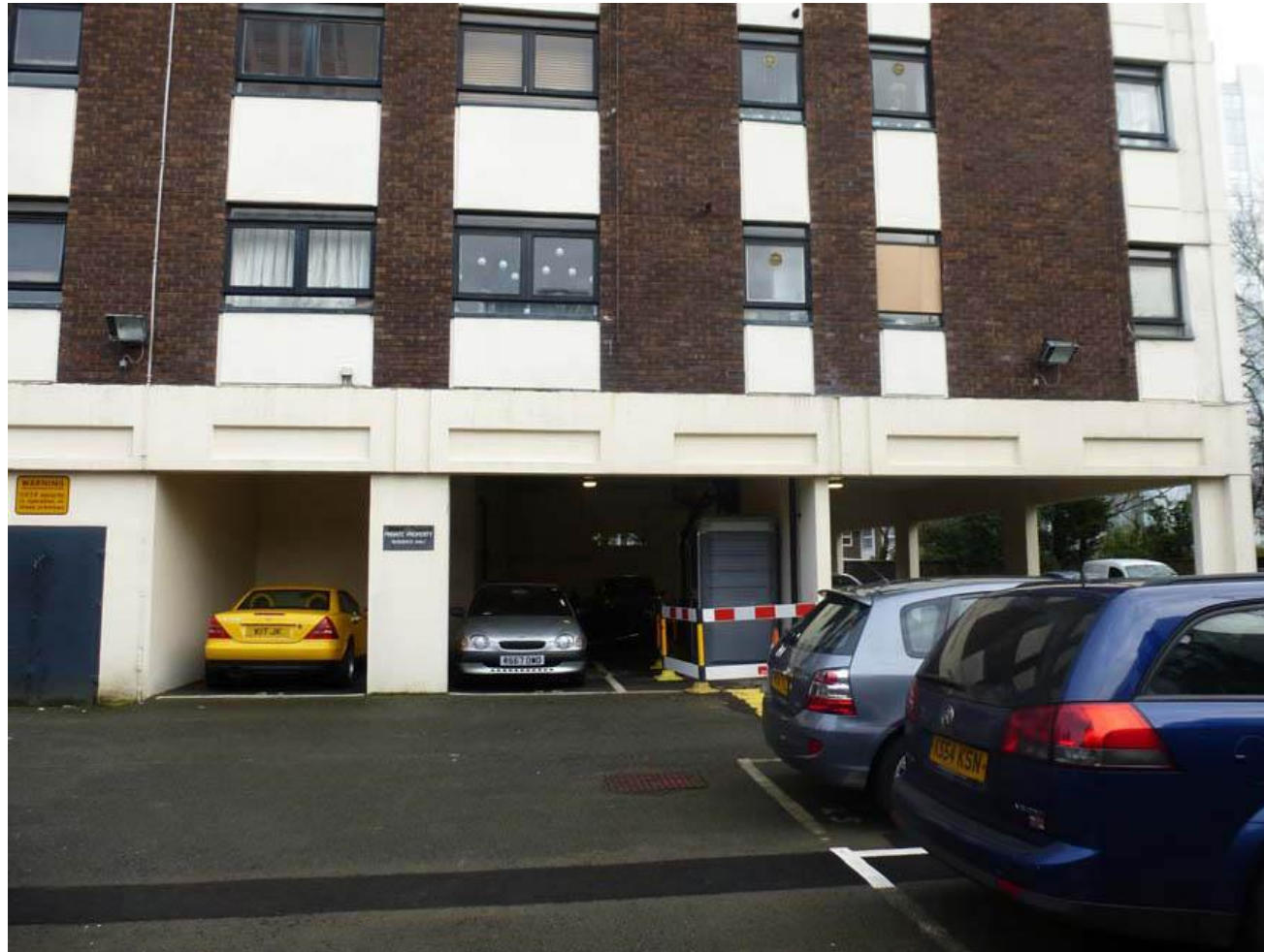
Undercroft, Kings College Court
