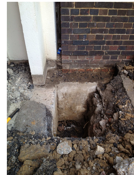
Figure 7: Example of trial pit
