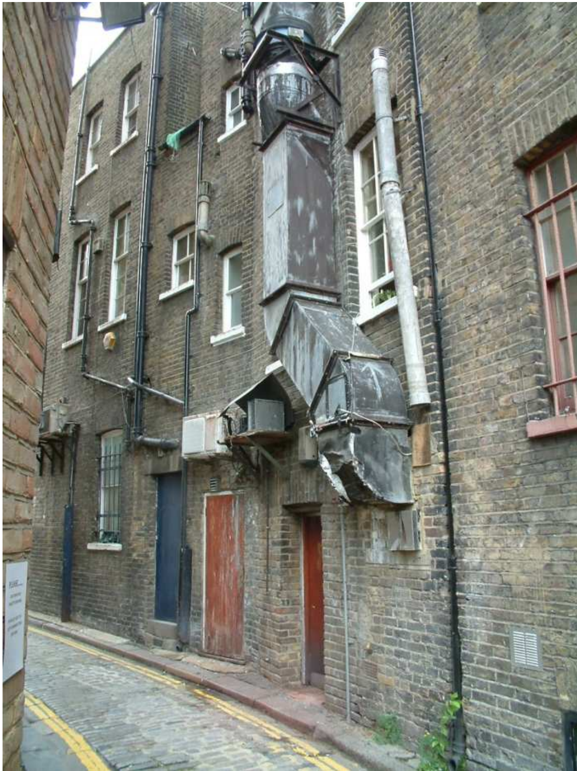
Photograph 1 Bird in Hand Yard before Occupation of Unit by Trevor Sorbie, showing previous air conditioning units and the large extractor ductwork.
