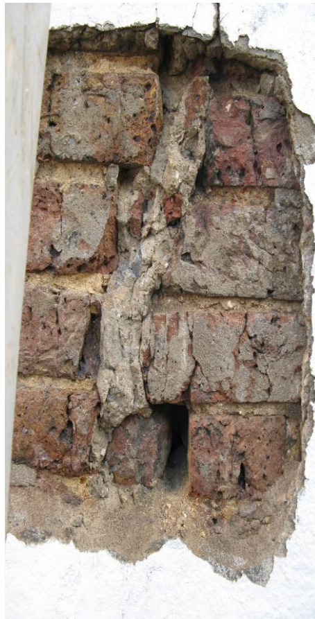
PHOTOGRAPH 4 Masonry fracturing
