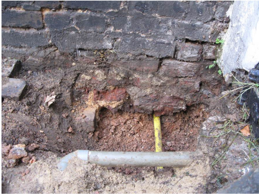
PHOTOGRAPH 3 Dilapidated brickwork
