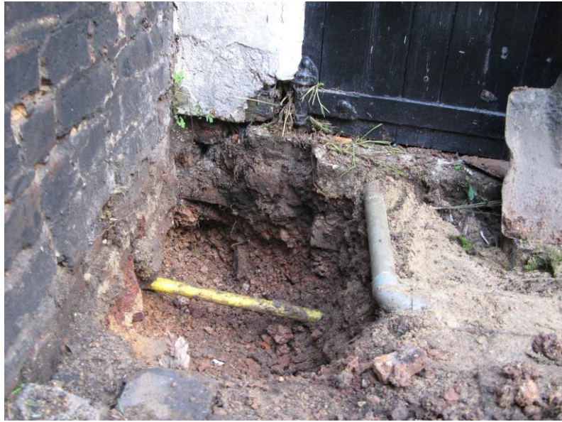
PHOTOGRAPH 5 Displaced dilapidated brickwork
