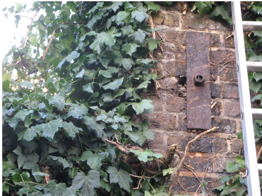
PHOTOGRAPH 2 Tie bar end, South East end
