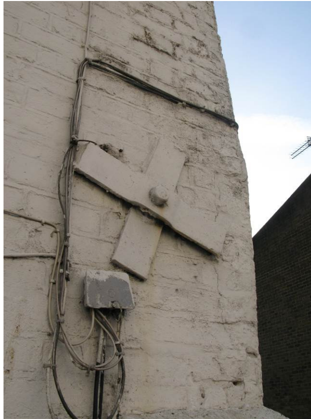
PHOTOGRAPH 1 Tie bar end, North West end
