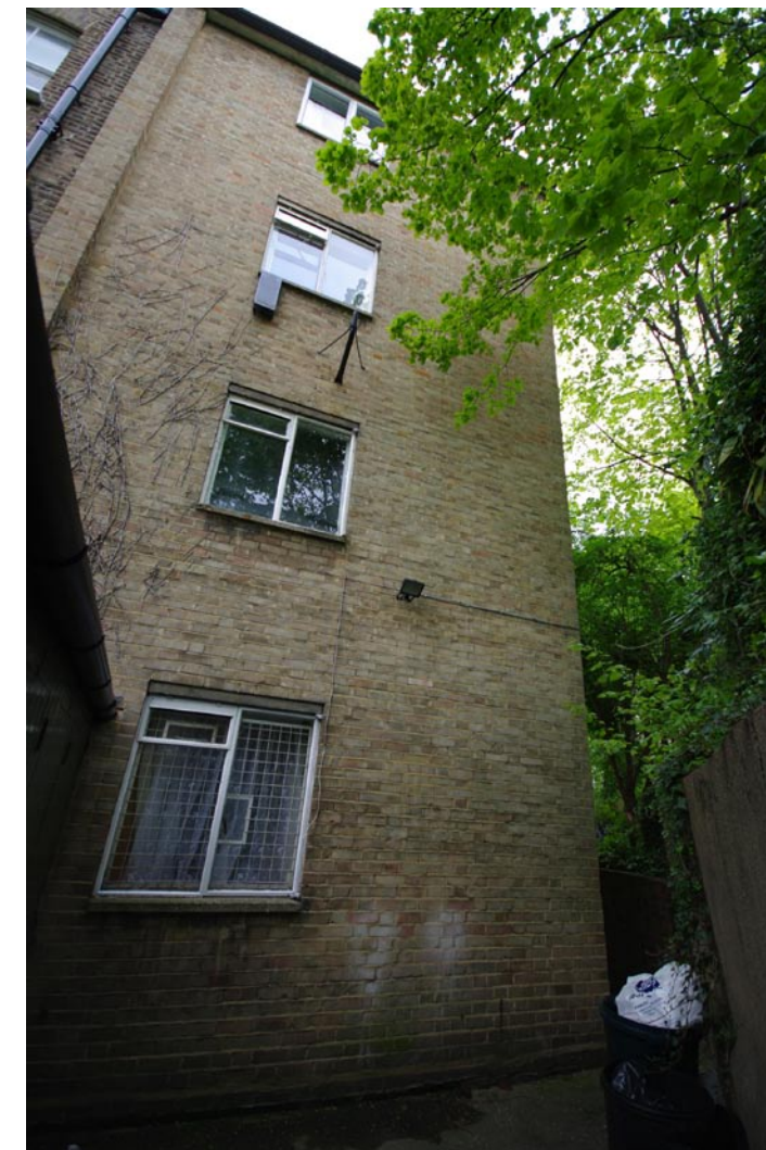
The existing bedroom windows located on the east facade facing the gardens of Brecknock Road. The original windows and doors are W20 Crittall windows with fine steel frames.
