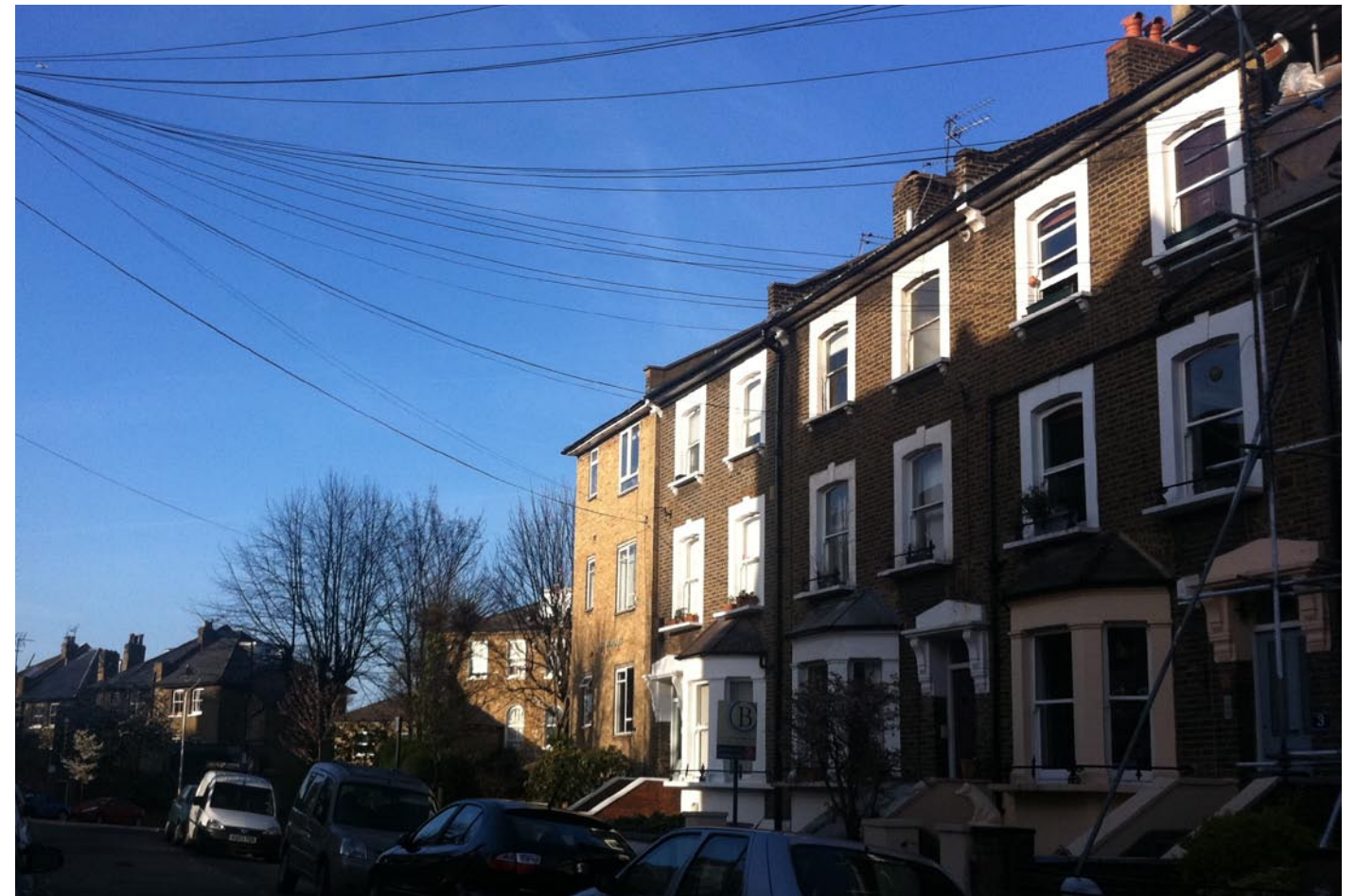
The Poplars building was designed to fit in as another house in the terrace, a brick building the same width as adjoining properties. It is clad in buff coloured brick and has a pitched roof consistent with its neighbours. Windows to the living rooms and kitchens of each flat are arranged in a pattern similar to the houses next door.
