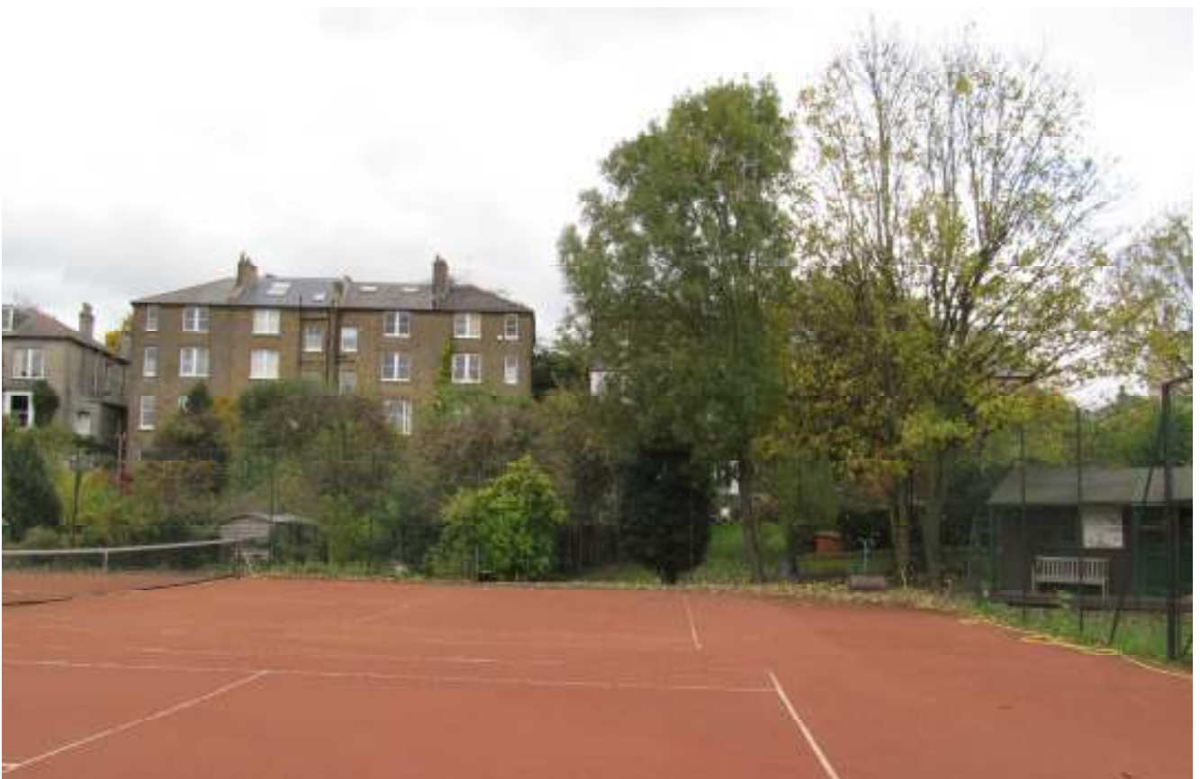
Photo 2 Rear gardens of houses to Dartmouth Park Avenue Note 1 No evidence of movement to rear elevations
