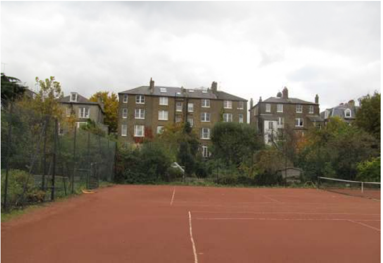
Photo 1 Rear gardens of houses to Dartmouth Park Avenue Note 1 No evidence of movement in rear elevations
