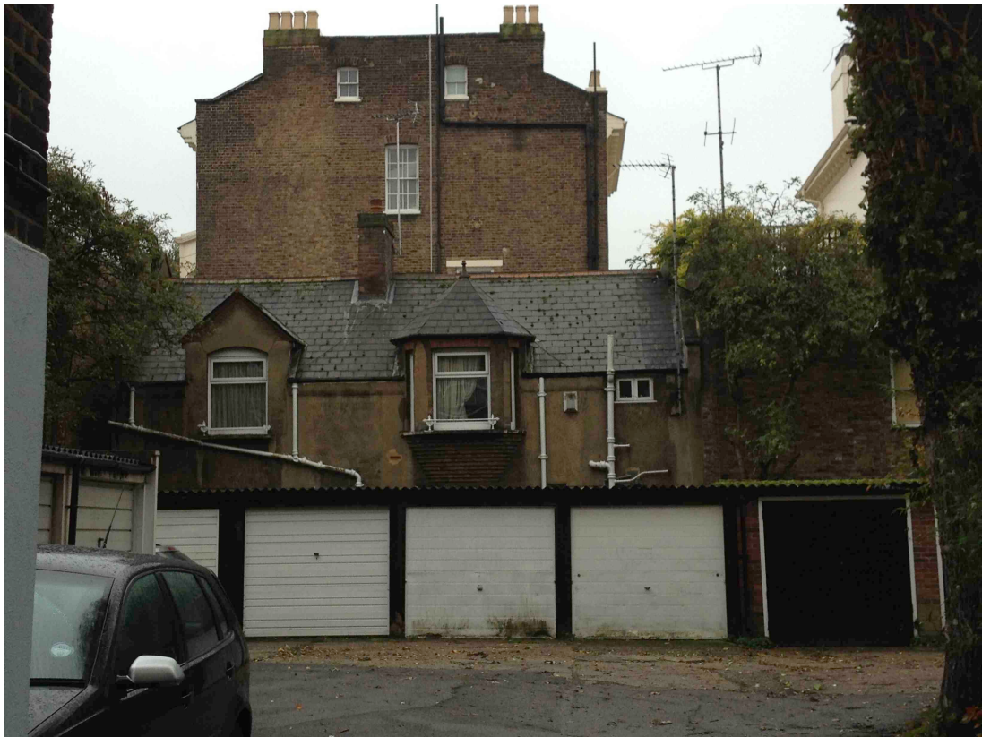
REAR ELEVATION FROM CAR PARK TO no.9 GLOUCESTER AVENUE
