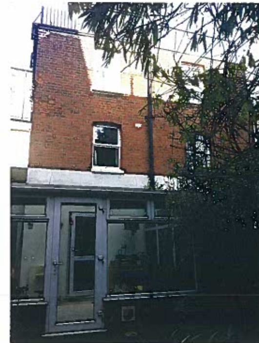
3 REAR ELEVATION OF 2B AND 4 HILLFIELD ROAD
