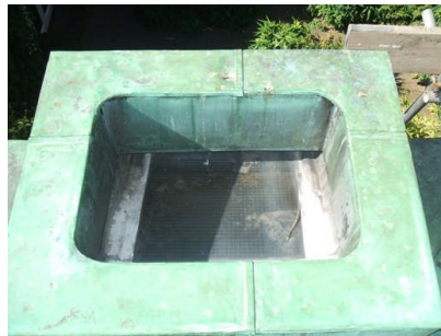
Roof skylights to be removed and reformed
