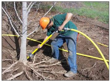
Photo showing root investigation work utilising an air spade
