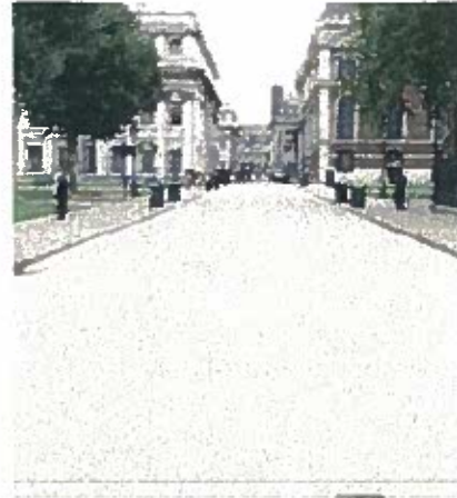
Bound gravel in the Street
