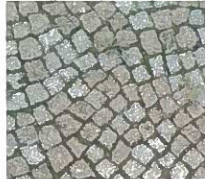
Cube setts in Mews Courtyard
