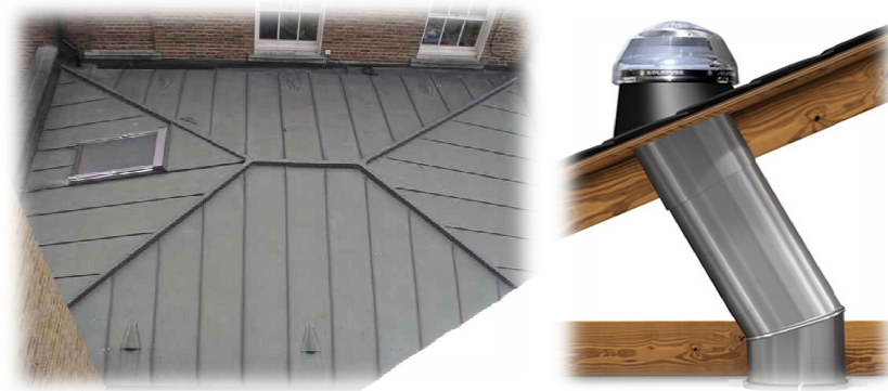
FIGURE: Photograph showing the existing roof covering and sky light and a typical section showing the installation of a sun pipe.
