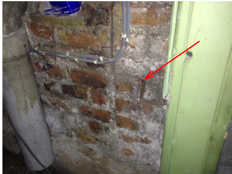
Figure 5 Cracked rear Wall
