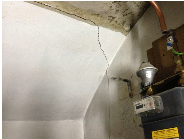
Figure 2 Cracking to Front Vault
