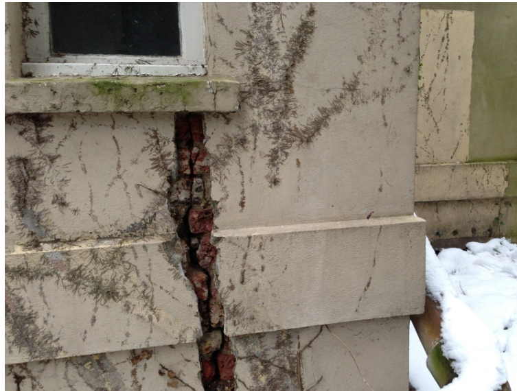
Figure 4 Cracking to Rear Side Corner
