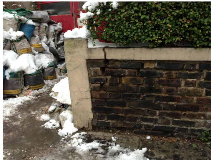
Figure 1 Front Wall Damage by Tree
