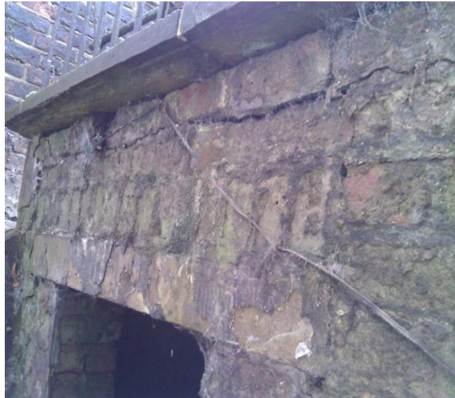
Photograph #4: Cracking of the brickwork under the coping stones which support the railings on top of the vaults. Also, shows the very limited depth available to the lime tree growing above the vaults.
