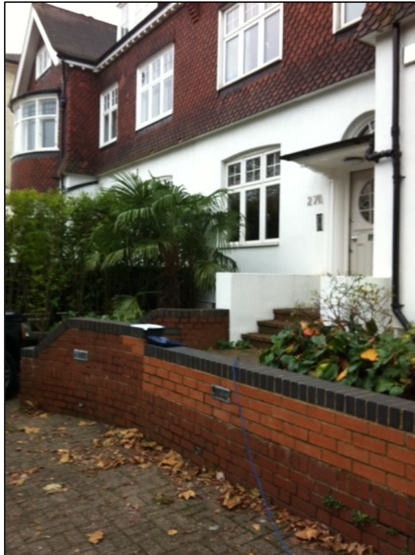
3 Raised entrance, weep holes visible.
