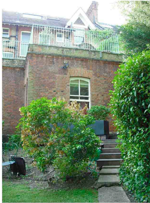
PHOTOGRAPH 2: REAR WINDOW SEEN FROM GARDEN
