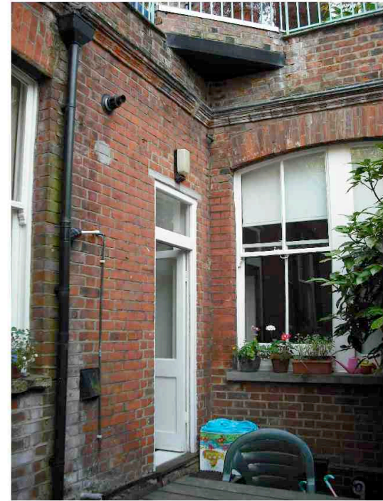
PHOTOGRAPH 3: EXISTING GARDEN DOOR
