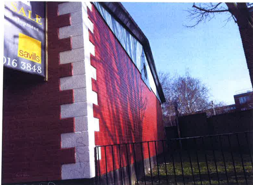
Print 2 – View of the south of the site area
