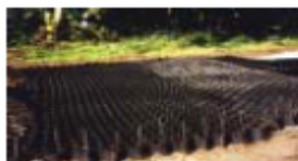
Expanding and staking Geoweb panels
