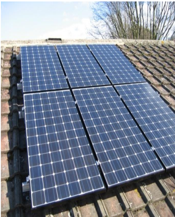
Photo-Voltaic Array
