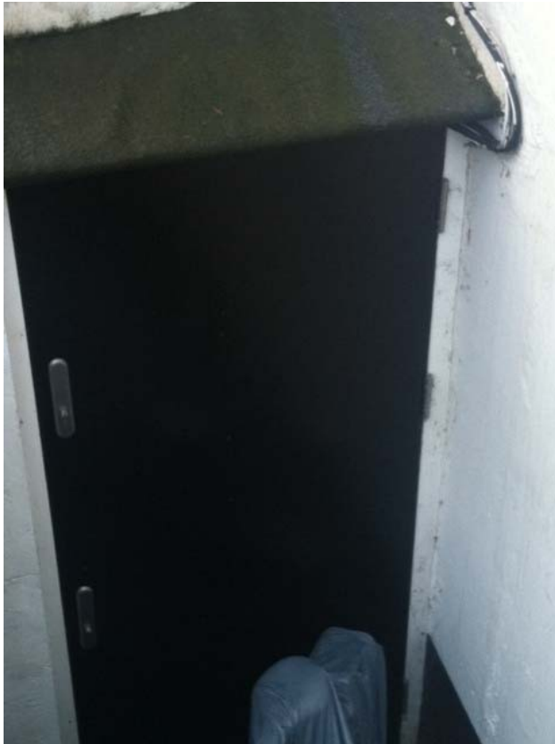
Existing basement door (from outside)
