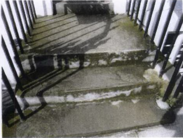
Existing front steps
