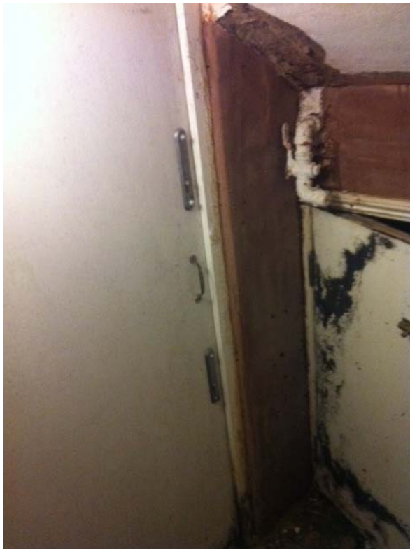
Existing Basement Door (from inside)
