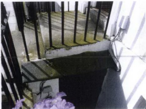
Existing roof over basement door
